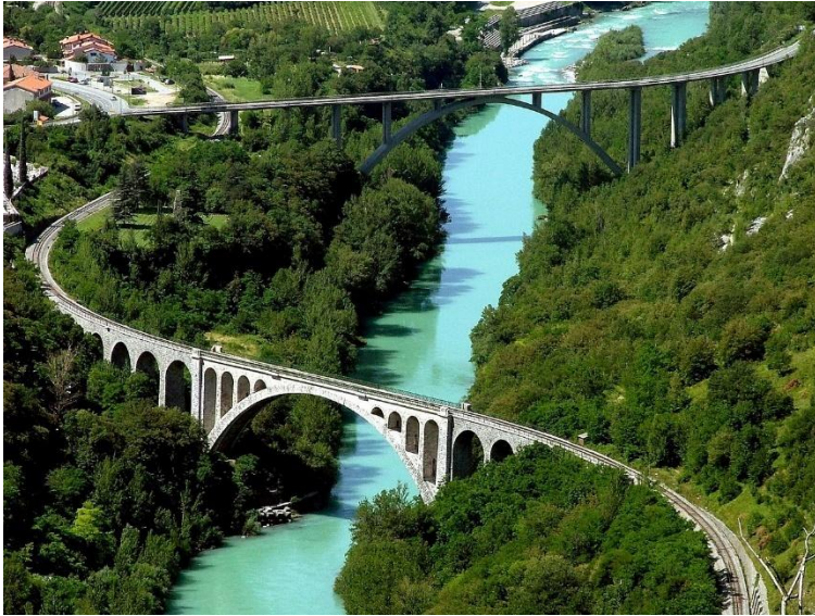
Solkan Bridge over the River Soča on the Bohinj Railway 66
