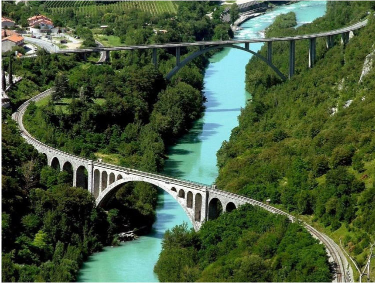
Solkan Bridge over the River Soča on the Bohinj Railway 71
