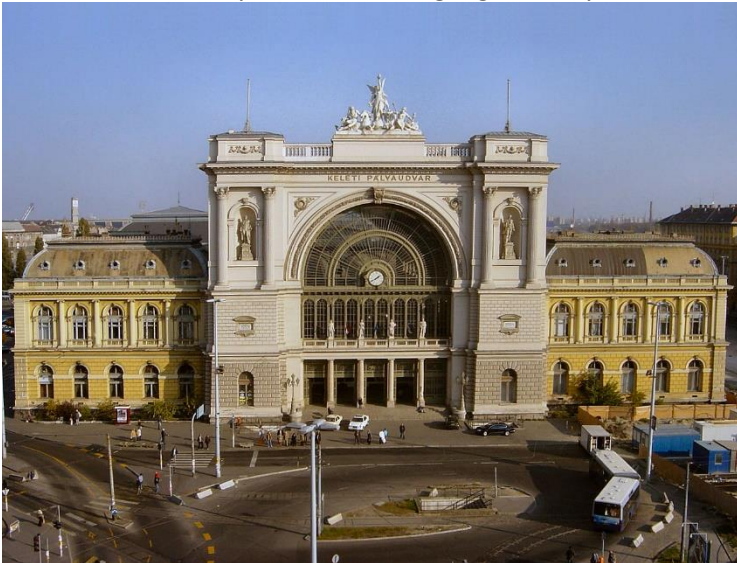
Budapest Keleti (east) railway station designed by Gyula Rochlitz and János Feketeházy and constructed between 1881 and 1884 39
