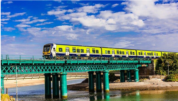
A CIE commuter service crosses Laytown viaduct, County Meath 44
