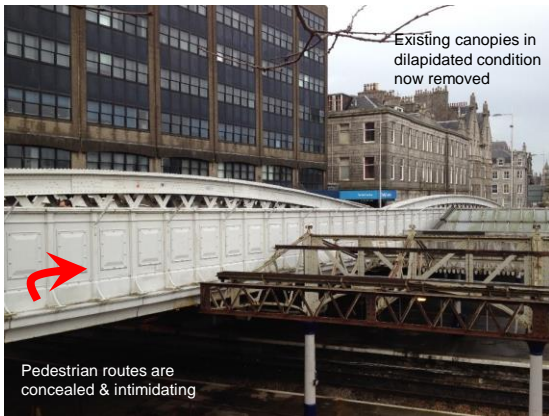
View of bridge looking Northeast towards Atholl House
