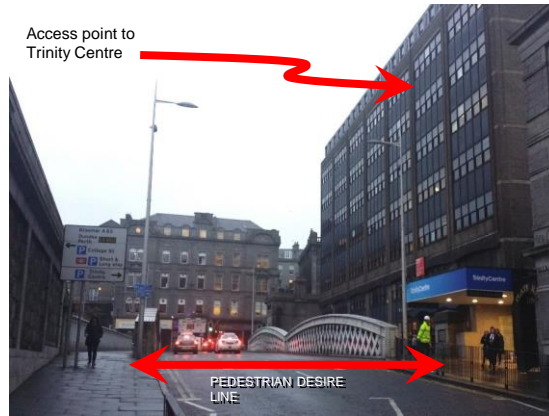
View of bridge looking West towards Bridge Street
